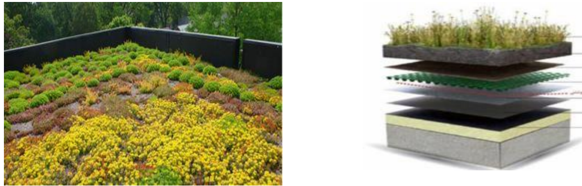
Figure 5. Natural insulation of a roof in regenerative design
